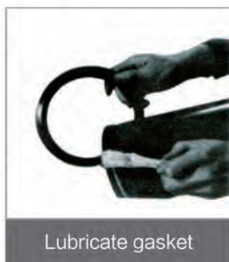
Gasket installation
