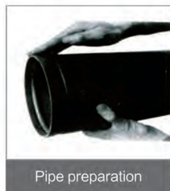
Lubricate gasket
